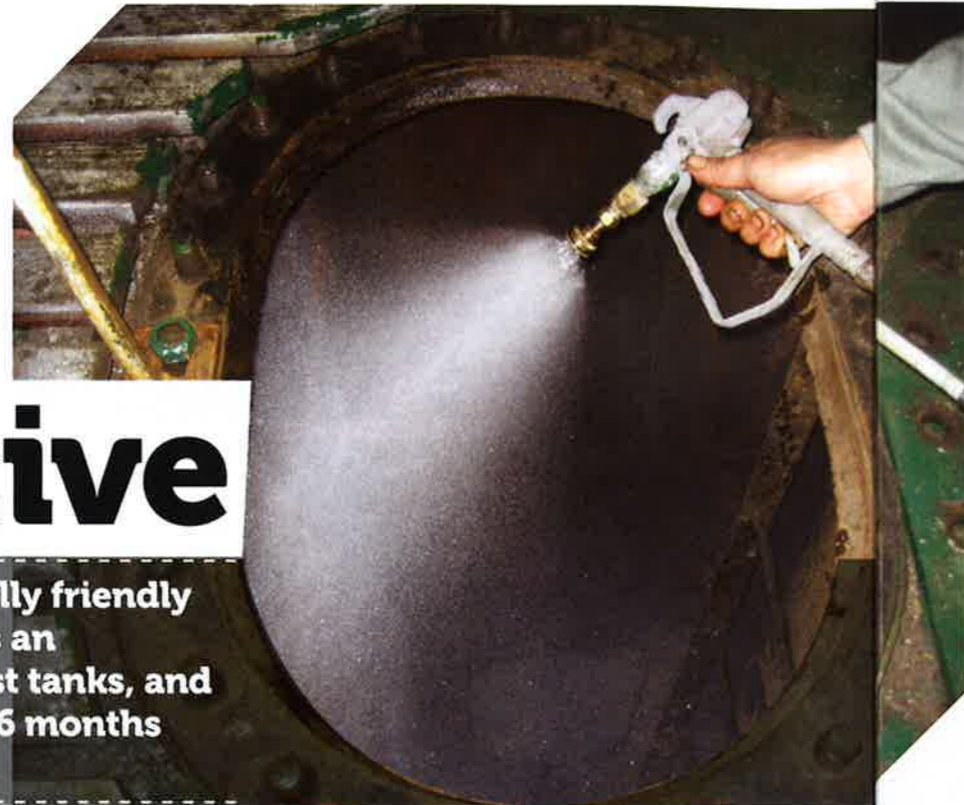
ABOVE: Taken after treatment, CSR I can offer protection for steel surfaces for up to 18 months
