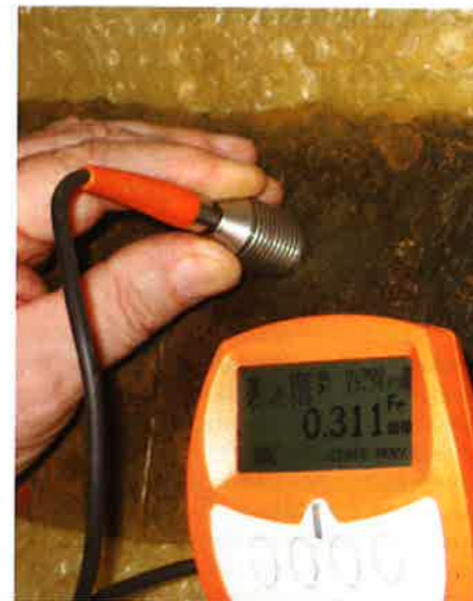
ABOVE: Step test panel for old rust and scale removal by micron
